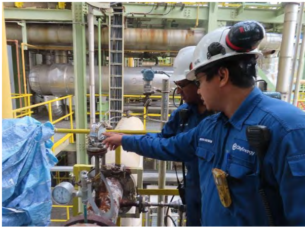
Pneumatic Pressure Test
