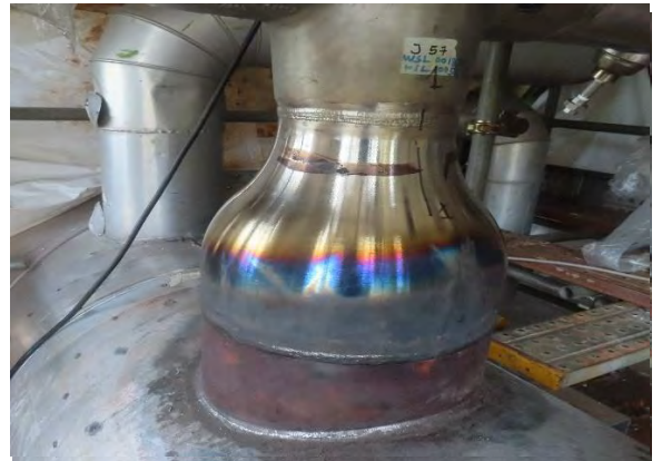
Gas Chamber Nozzle Installation
