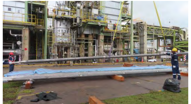
Lifting & Installation of New Reformer Tube
