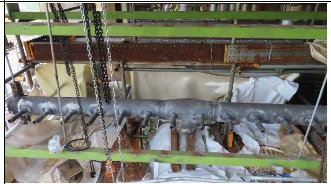
Demolition of Gas Chamber Manifolds
