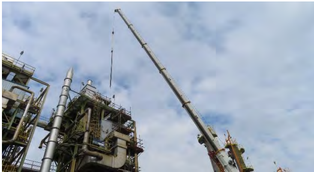
Lifting & Removal of Existing Reformer Tubes
