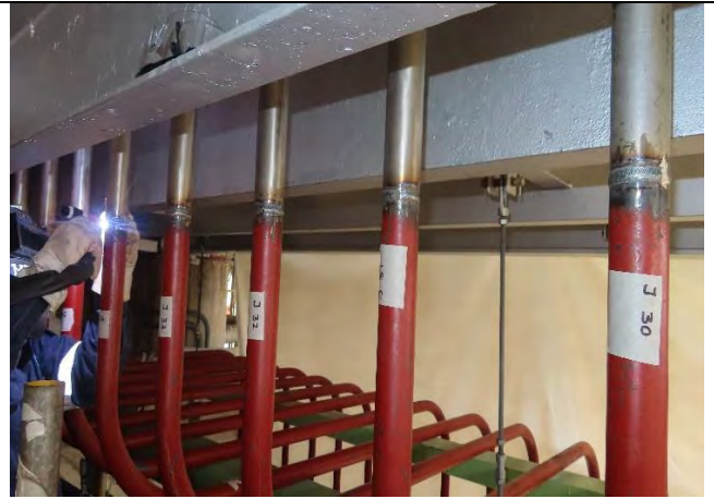
Welding Of Inconel Piping
