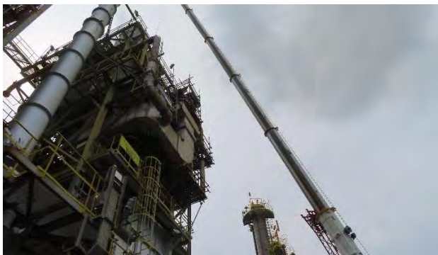
Removal Of Existing Reformer Tubes by Crane
